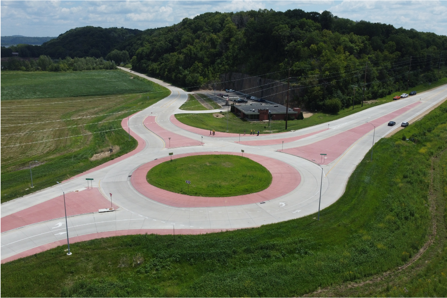
FIGURE 11.4 BUILD Grant Improvements - John Deere RD Source: Dubuque County
